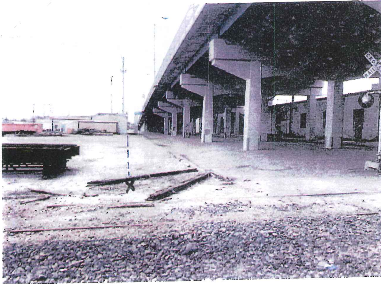
LOOKING NORTH ALONE BETWEEN EAST
